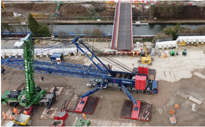
— Spreading the Load from Outriggers
