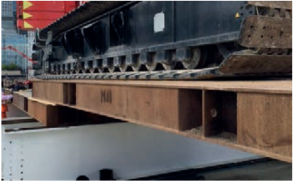
— 250t Crawler on Steel Mat Bridge
