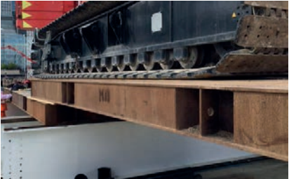
→ 250t Crawler on Steel Mat Bridge
